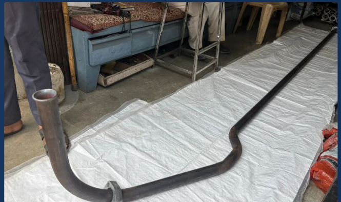
Pipe bending and custom fabrication
